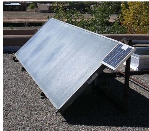
One solar hot water panel like this provides enough solar heat to heat up one 80-gallon water tank each day in New Mexico - about enough for the average family to take showers and wash the dishes once.
