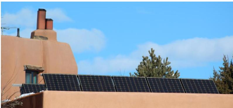
elements are designed for. The two rows of panels are connected in parallel, so the voltage is still 250 Volts at the water heater. It was easy for our solar installer to run the wires in conduit from the south roof to the inconvenient utility room on the north side of the house. It only took part of a day to remove the old water
