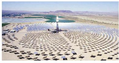
"Solar II" was tested in California, but its technology was first invented and tested in New Mexico, at a National Laboratory in Albuquerque (Sandia National Labs). Solar II could actually store the solar heat using "molten salt", which was used to smooth out the output of the plant, and keep it going when clouds passed by. The tanks of molten salt can be seen in the photo on either side of the base of the tower.
