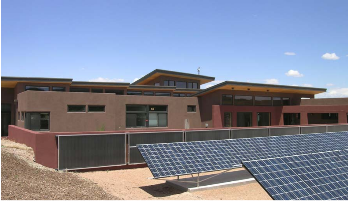
VIEW OF OLSEN RESIDENCE FROM SOUTHWEST
